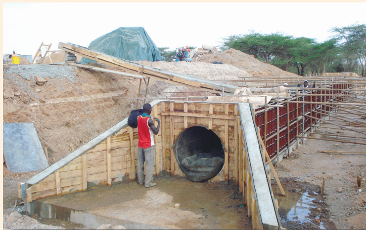
A section of the Isiolo-Marsabit road currently (2008) under construction
