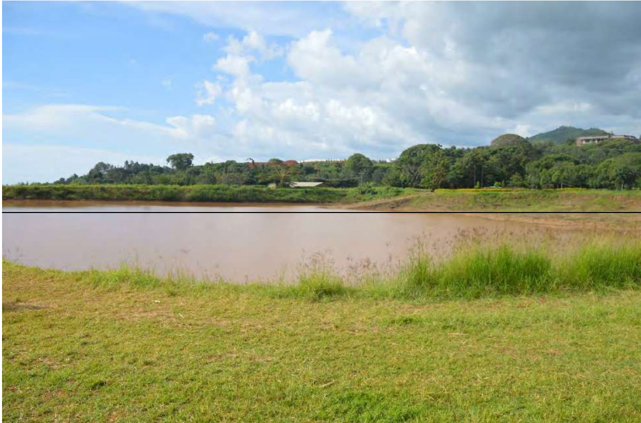
One of the dams within the Patel Coffee Estate in Solai, Nakuru.
