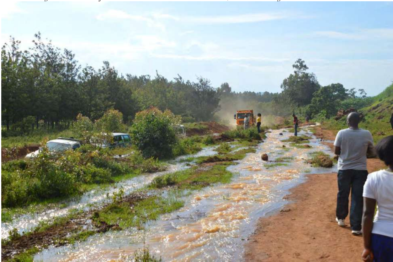
Water from one of the Patel dams discharged by government officials, flowing on the main road, into people’s farms and causing further damage.
