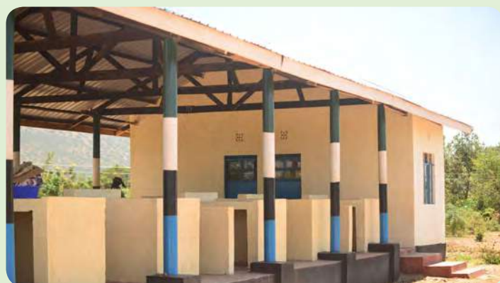
One of the newly constructed markets
