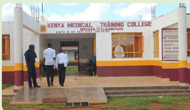
The newly constructed KMTc, Busia
