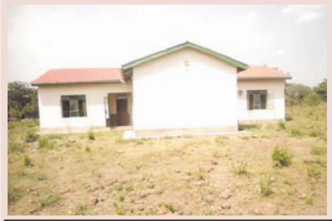
Cherwa dispensary in Nyakach Constituency constructed using CDF but is not operational owing to lack of staff and equipment
